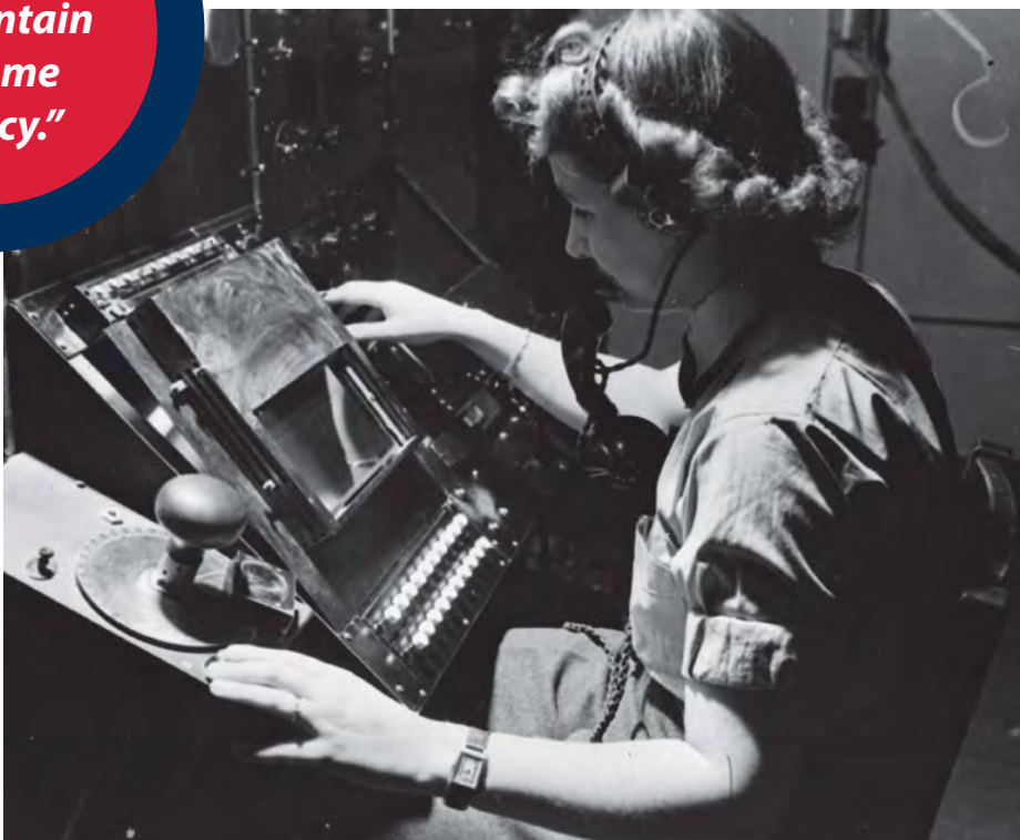
Right: WAAF radar operator Denise Miley plotting aircraft on the cathode ray tube of an RF7 receiver in the receiver room at Bawdsey CH. Her right hand has selected the direction or height-finding and her left hand is ready to register the goniometer setting to the calculator. May, 1945.
