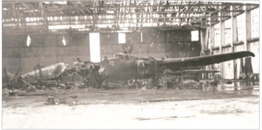
Above, Damage at RAF Driffield, 15 August 1940
