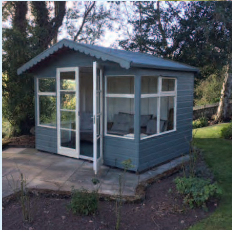
Rothbury House refurbished summer house
