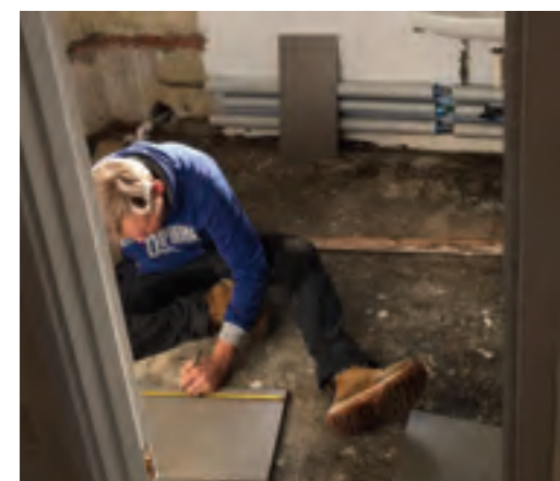
Still got it: Putting plumbing and tiling skills to use © MOD/Crown
