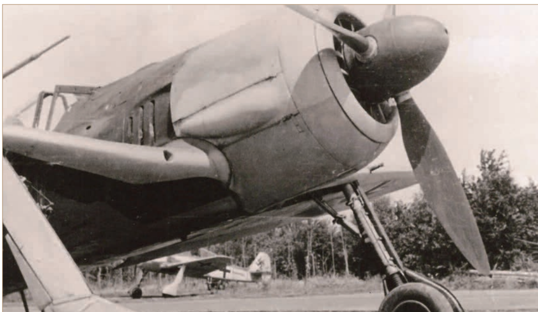
A good view of the radial engine cowling. Photo: © Author
